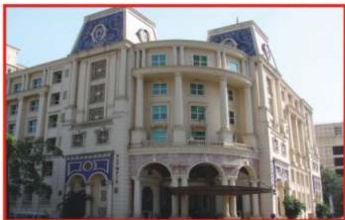
OLYMPIA M/S. HIRANANDANI CONSTRUCTIONS
