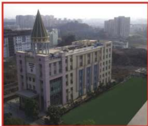
NEW SCHOOL, POWAI-M/S. HIRANANDANI CONSTRUCTIONS
