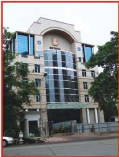
BRITISH GAS HOUSE M/S. HIRANANOANI CONSTRUCTIONS
